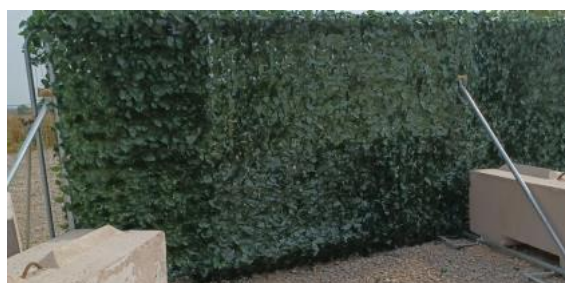
Plate 3.4 Herras fencing with attached textured plastic hedgerow (source: HS2/ EKFB, in Reason, P.F. and Wray, S. (2023). UK Bat Mitigation Guidelines: a guide to impact assessment, mitigation and compensation for developments affecting bats. Version 1.1. Charter
